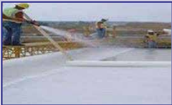
Fig 6 - Curing of concrete
