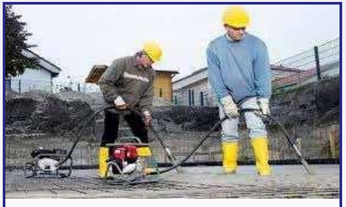
Fig 5 - Compaction of Concrete
