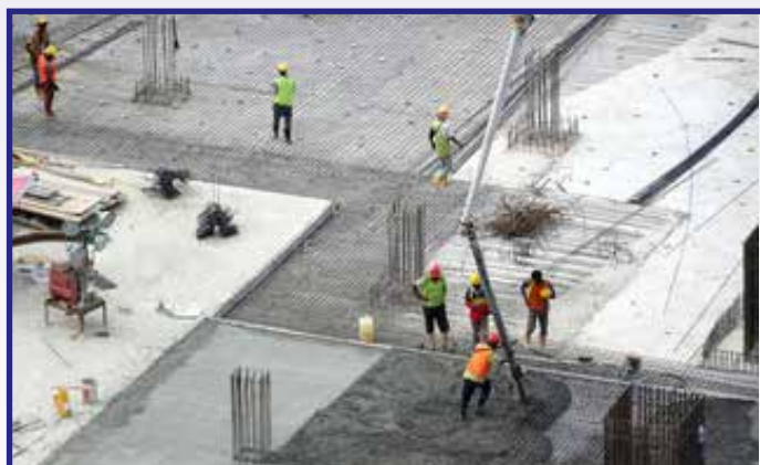
Fig 8 - Placing of concrete
