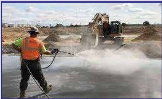
Fig 10 - Curing of concrete
